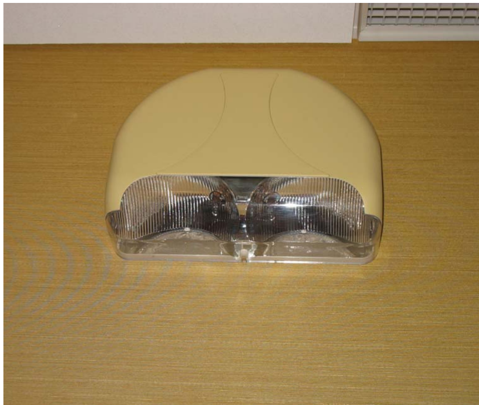
Figure 2: Emergency Lighting (Typical)
