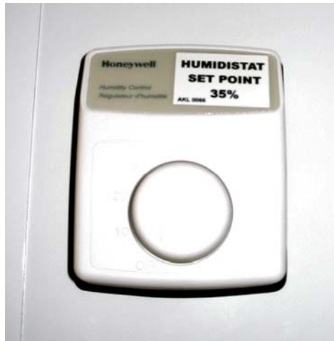
Figure 32: Humidity Controller
