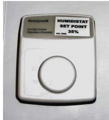
Figure 37: Humidistat Control
