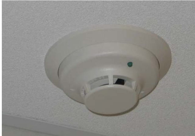
Figure 18: Smoke Detector
