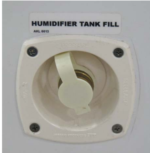
Figure 16: Fresh Water Connection
