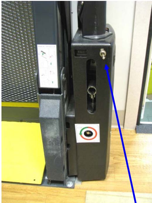
Main Power Switch
