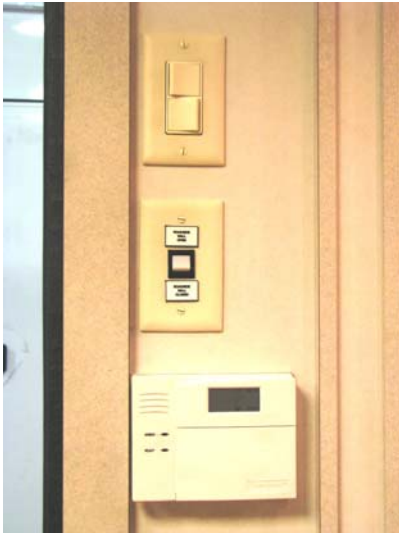
Lighting and Slide-out Controls and Intrusion Alarm Panel
