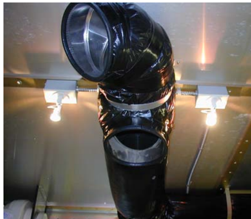
Magnet Room Lighting
