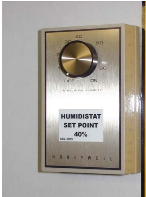
Figure 43: Humidity Controller
