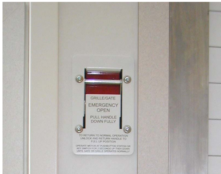
Figure 32: Roll Door Emergency Release
