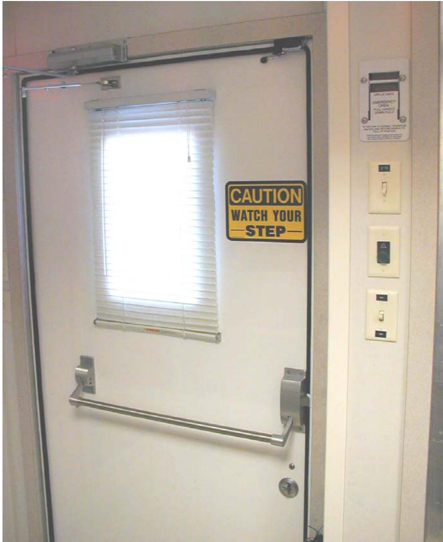
Figure 12: Exterior Staff Door
