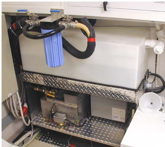
Figure 41: Humidifier (Typical)
