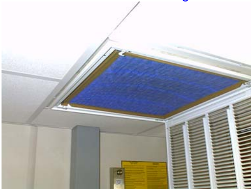
Downstream Blower Filter Access
