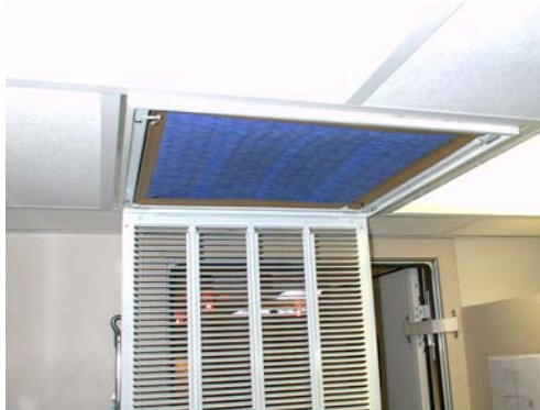
Downstream Blower Filter Access
