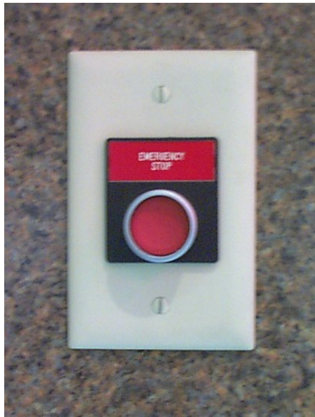
Figure 22: Emergency Shutdown Buttons
