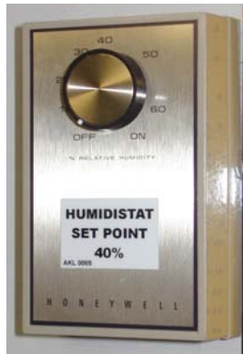
Figure 29: Humidity Controller
