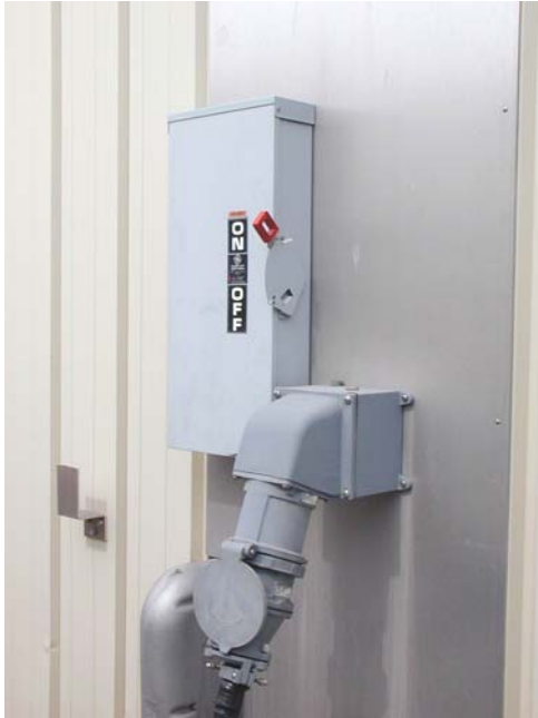
Figure 27: Shore Power Connection
