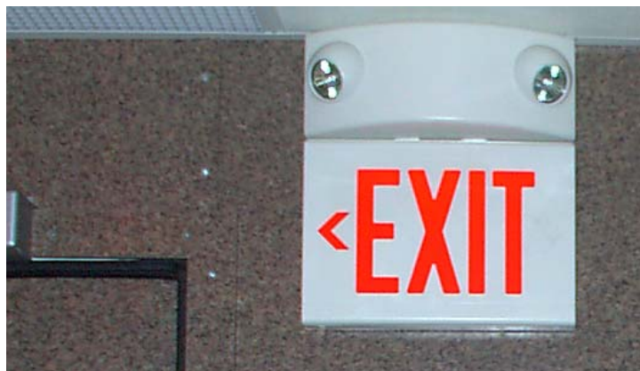
Figure 17: Emergency Lighting
