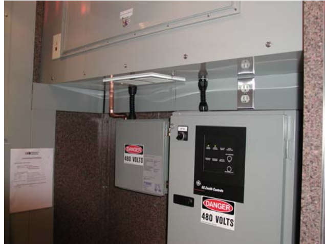
Figure 25: 480V and 120/208V AC Electrical Panels
