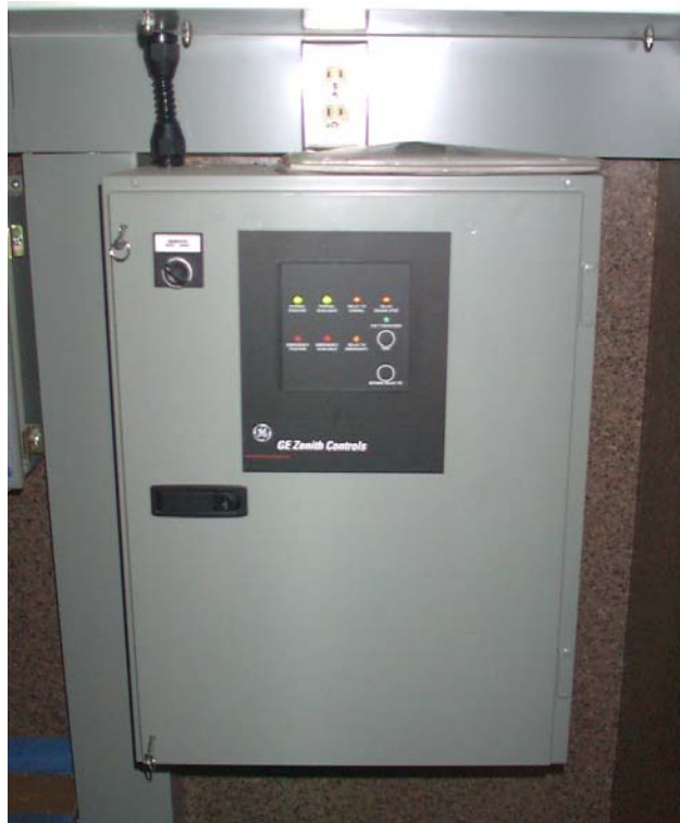
Figure 23: Automatic Transfer Switch
