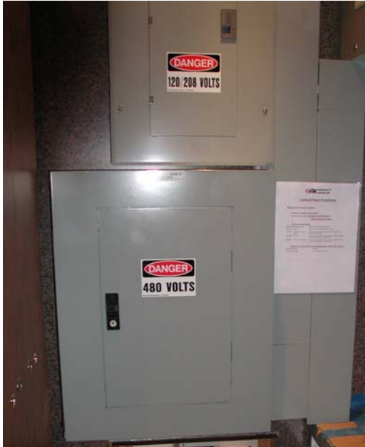
Figure 25: 480V and 120/208V AC Electrical Panels
